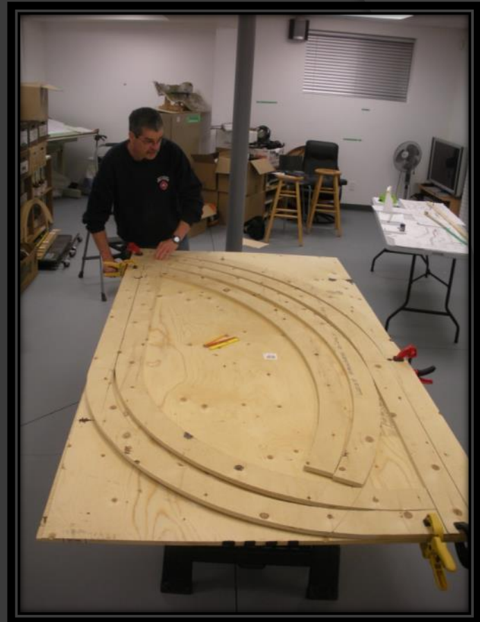
CONSTRUCTION OF CURVED DIVIDER WALLS
